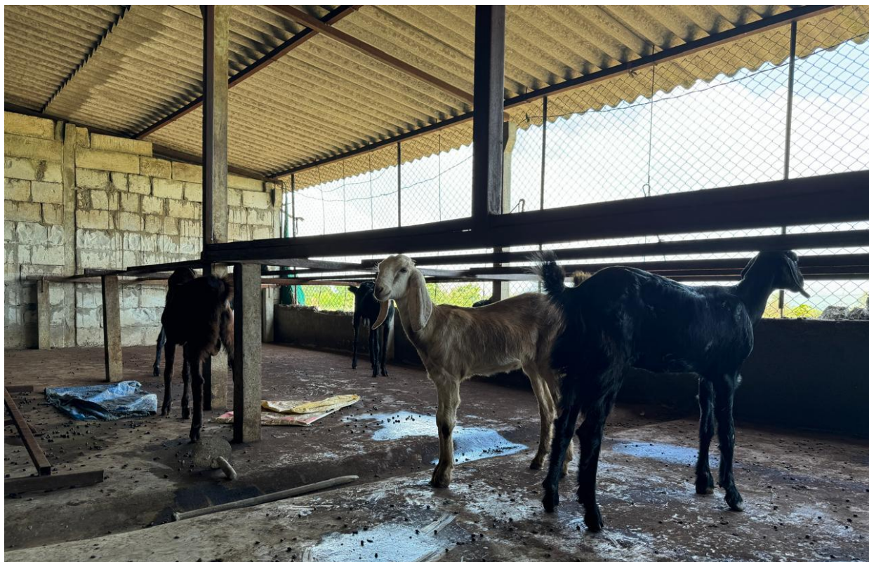
RCC goat shed constructed by a ST farmer, using the earnings through sale of goats
