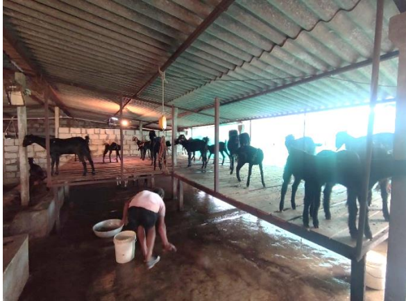
Newly constructed goat shed with GI sheet roof and concrete floor from earnings through selling of goats by a tribal farmer of Vinayaknagar village
