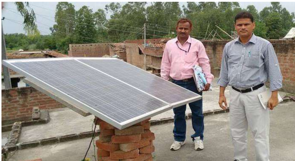
Solar panel installed by MRIDA (NGO) at Tahtajpur village
